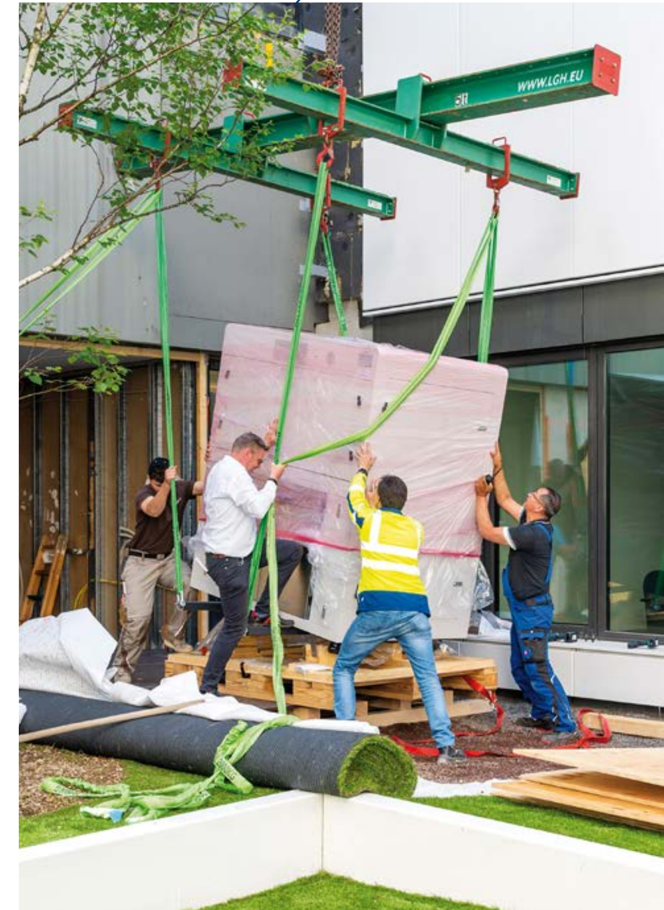
The 1.4-tonne printer would not fit through any door, and when it was delivered the front of the UKM building had to be opened up.
